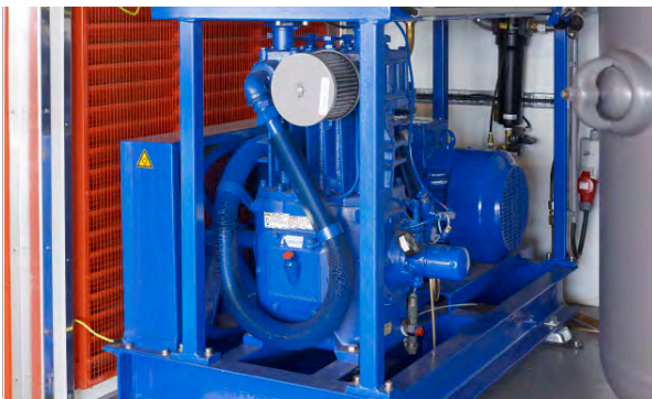
Low pressure compressor with a capacity of 1450 liter per minute at a pressure of 13 bar. This compressor is intended to operate the decompression chamber.
