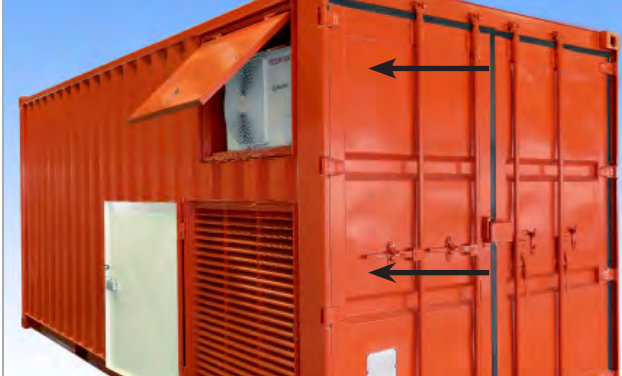
Air conditioner hatch above and the compressor hatch below.
