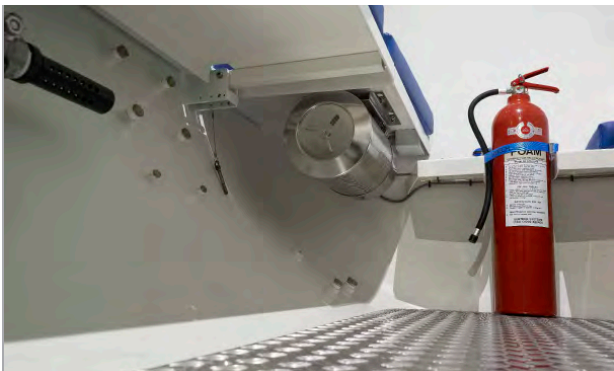
A fire extinguisher and a CO 2 scubber located inside the main chamber.
